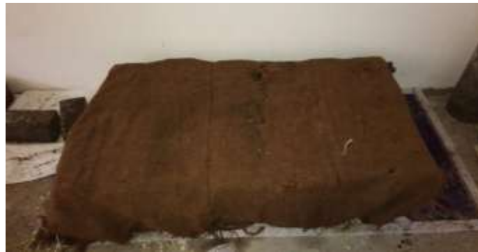
Fig no 3.5.1 Curing of blocks
