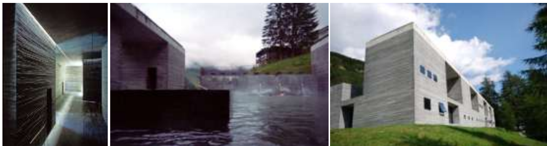
Figure 6.1.1/6.1.2/6.1.3 : The interior view; the outdoor pool; the exterior view
