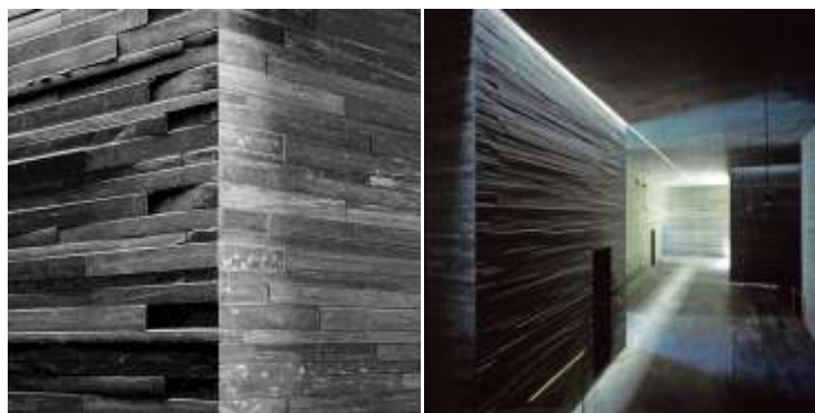
Figures 7.3.1/ 7.3.2 : Material finish as an element; Light as an element
