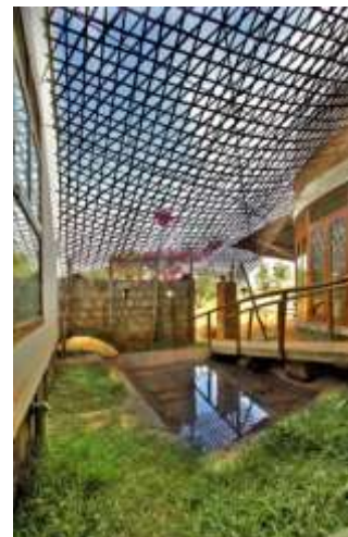
Figure 6.3.5: Bamboo roofing over pool
