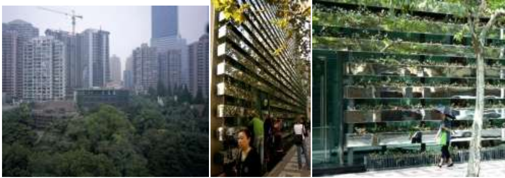
Figure 6.2.1 : Location of the building Figure 6.2.2/ 6.2.3 : Planters on the front facade
