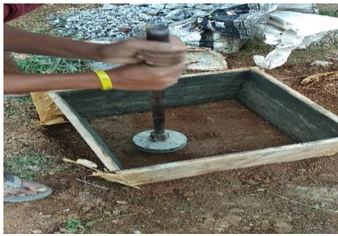
Figure -2: Subgrade preparation
