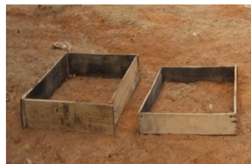
Figure -1: Moulds of prototype slab
