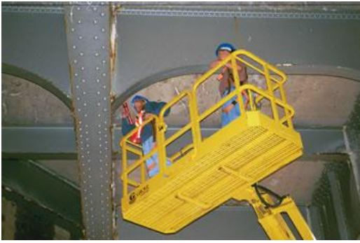
Figure 1.1 UT based visual inspection
