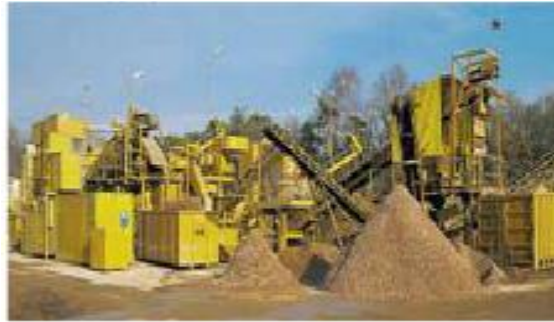
Aggregate crushing plant
