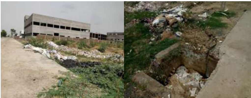
Fig -7: Solid waste disposed in vacant plots and side drains
