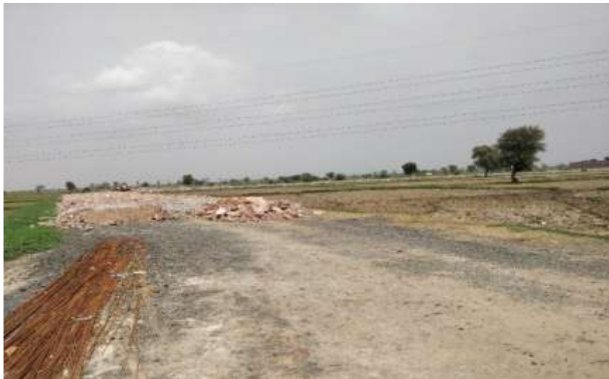
Fig -6: The road is being constructed by GIDC
