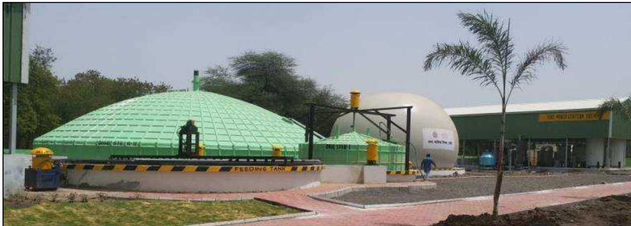
Figure 2 :- Biomethanation plant of organic waste in anaerobic digestion [Source:- Choithram mandi, Indore]
