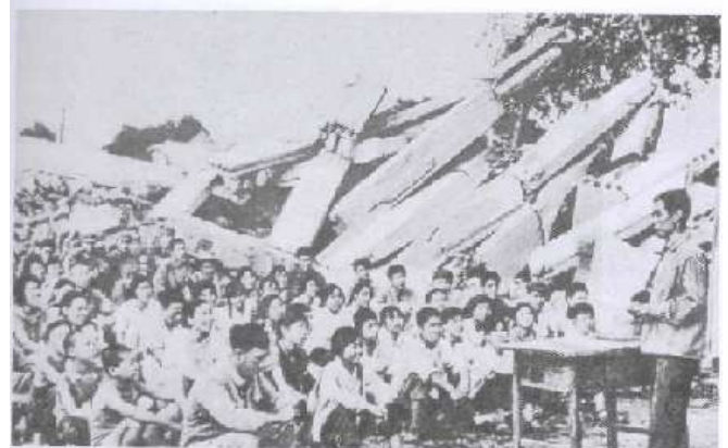
Fig 14 Collapse of precast buildings
