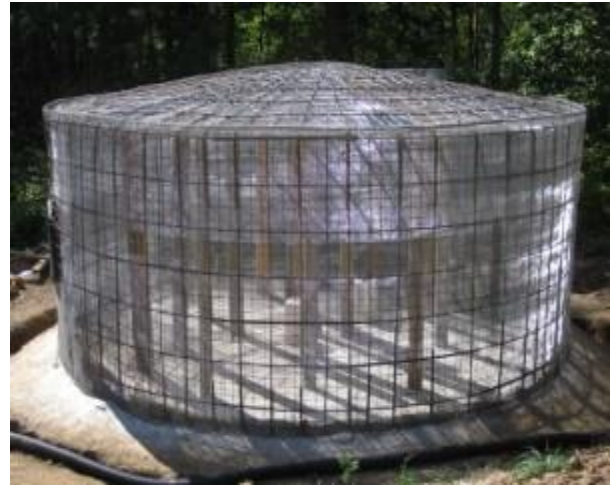
Fig-1: Ferro cement water tank
