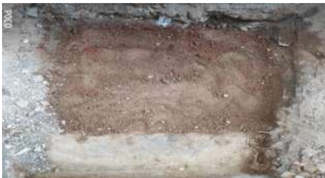
Fig 7.1 Excavation of soil
