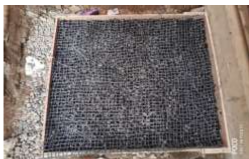
Fig 7.9 Laid geogrid in DBC layer
