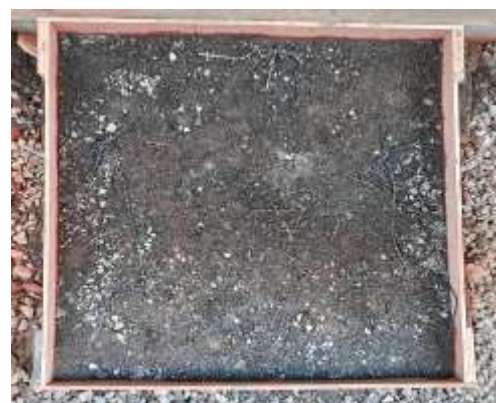
Fig 7.4 Geogrid laid in WMM layer
