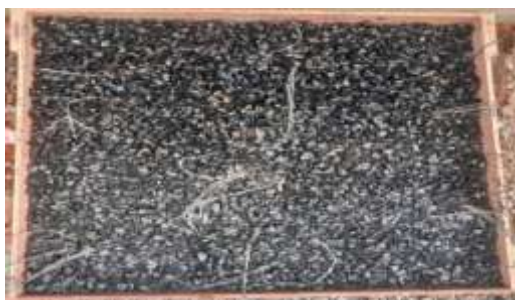
Fig 7.8 Before laying the geogrid
