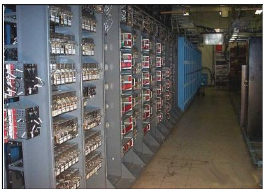
Image 2: Route Relay Interlocking.
