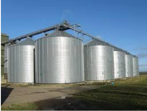
Fig -1: Flat Bottom Silos
