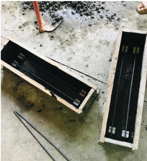
Fig 3.2: Casting of beams
