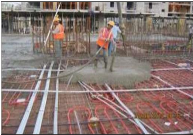
Figure: 4 Radiant Cooling Slab
