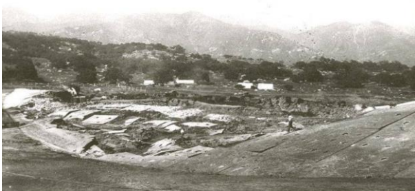
Flow Failure Liquefaction
