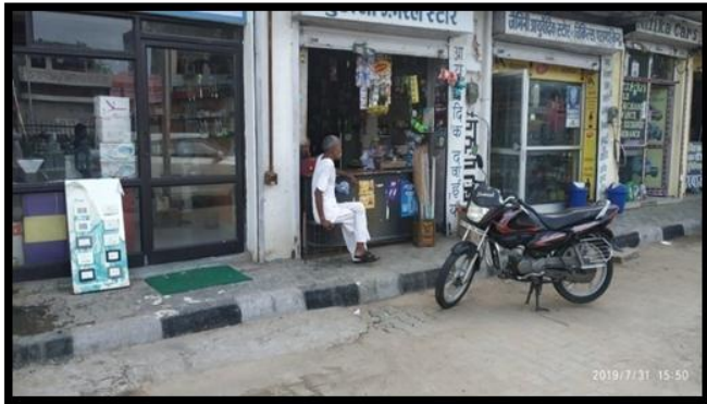
Fig – 9 Insufficient Width of Footpath
