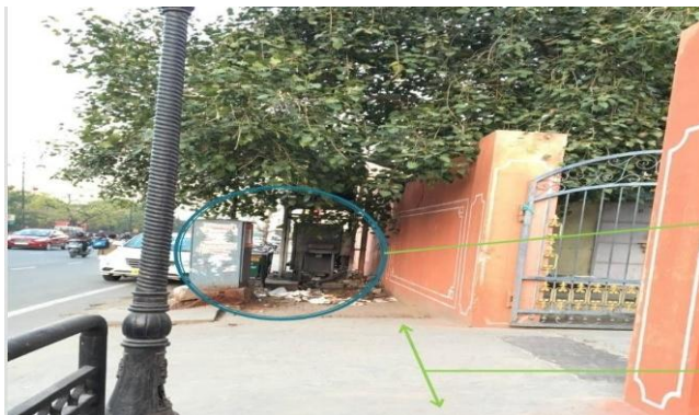
Fig - 4 Electric Boxed, Trees and Ramps on Footpath
