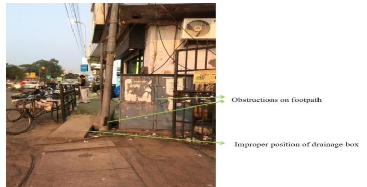
Fig - 6 Obstructions on Footpath
