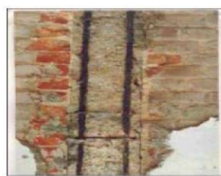
Fig No3 -Corrosion of Reinforcement
