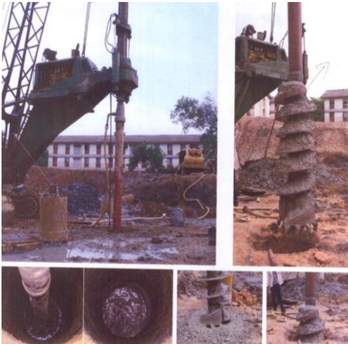
Figure 1. Boreholes at Different Locations
