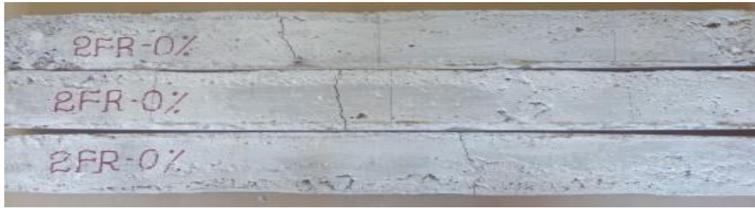
Fig 7: 2 layered flexural repeated beam ( V_f=0\% )
