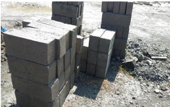
Fig -3: Curing and Placing of Blocks
