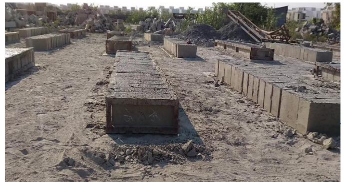
Fig -2: Casting of Mould
