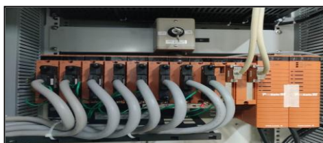
Fig.4.5: Node Unit of the controller with Pre-Fab cables connected.
