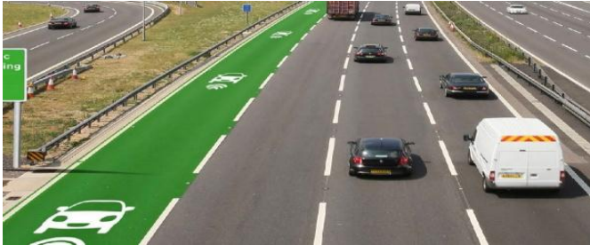
Fig1.2 A practical example of wireless charging of lane in UK.
