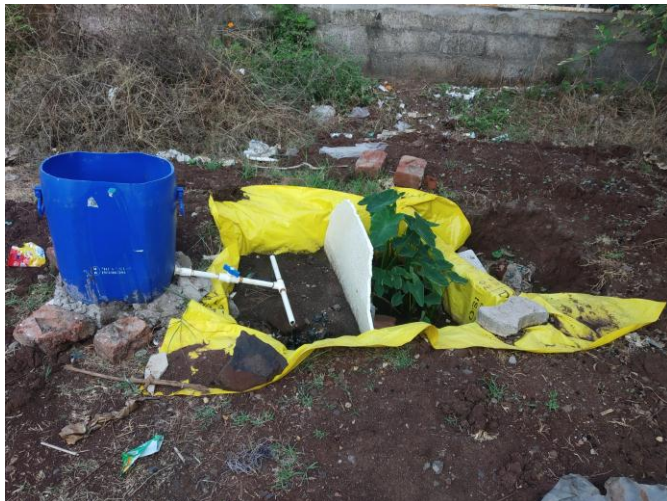
Fig-3: On site model of horizontal flow constructed wetland
