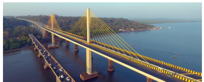
Fig -1: Cable Stayed Bridge, Goa
