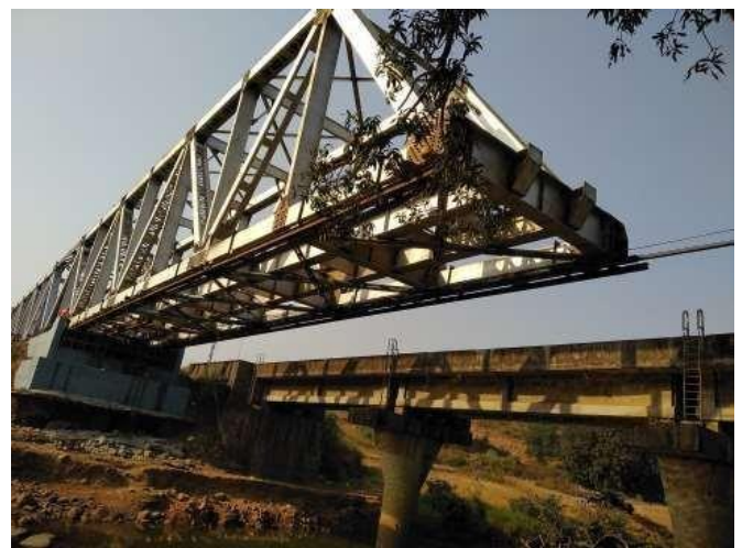
Fig-1: Launching of Bridge by Incremental Launching Method
