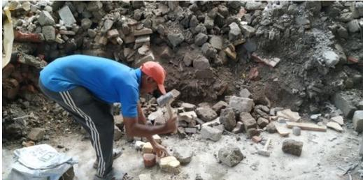
**Fig -3:** Manual Crushing
