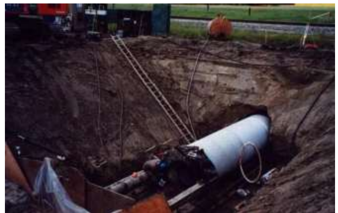
Fig -5: Pipe jacking method
