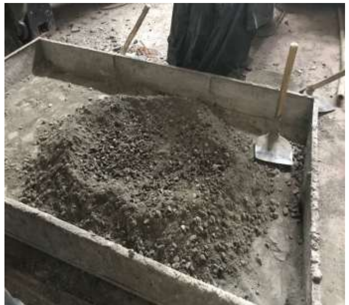
Fig. 6. Mixing of Concrete
