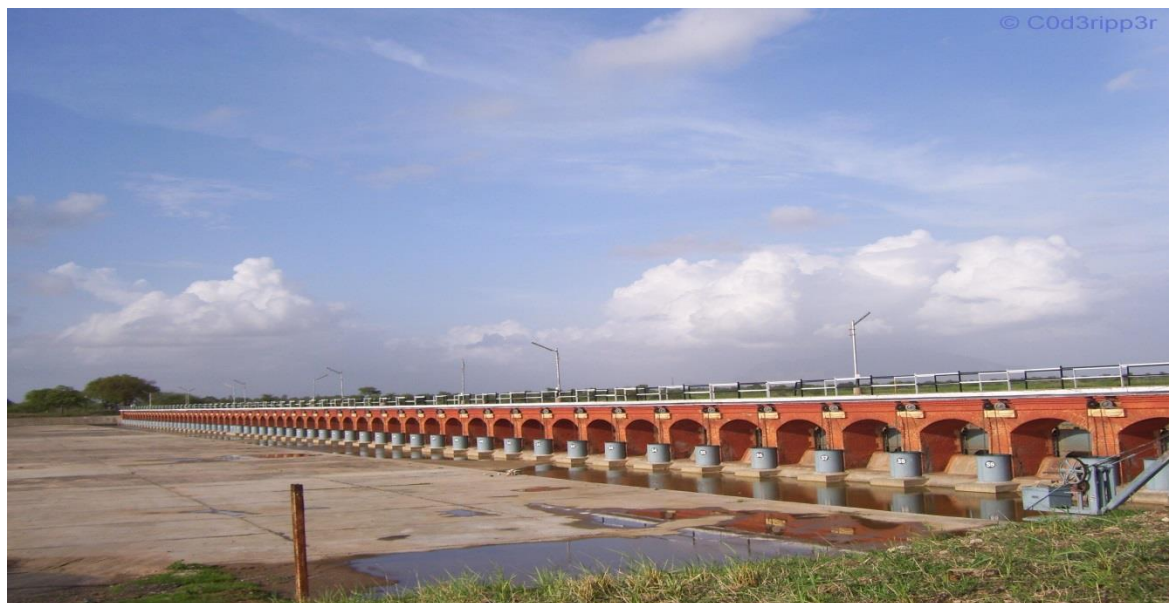
Figure 3 Ajwa dam on Vishwamitri River
