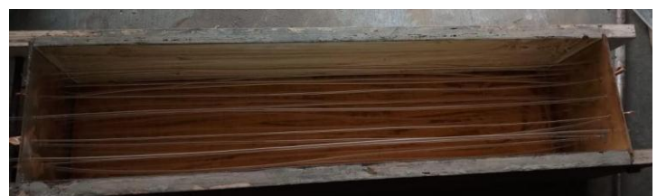
Fig 3.12: Mould with POF before pouring concrete in Beam
