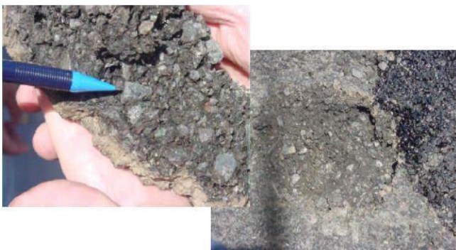
Figure 17. Stripping on road
