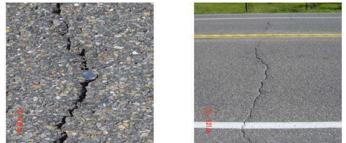
Figure 8. Transverse cracking on road
