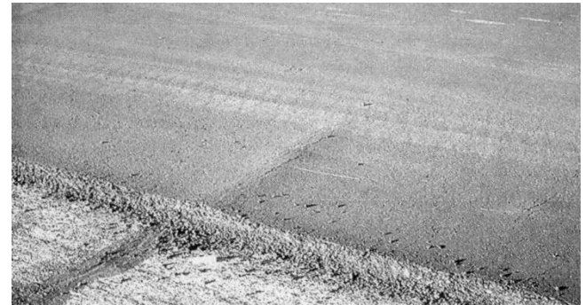
Figure 13. Overlay bumps on road
