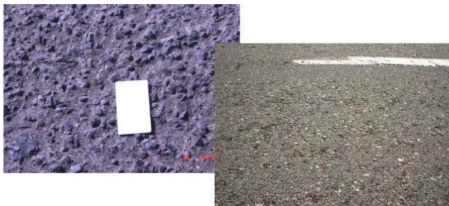
Figure 16. Ravelling on road
