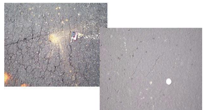
Figure 21. Checking on road
