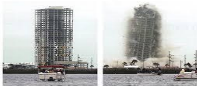
Fig – 7: Ocean Tower - Unfinished & Controlled
