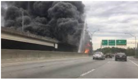
Fig - 11: Collapse of Bridge in I-85
