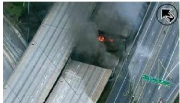
Fig – 9: Collapse of Bridge in I-85
