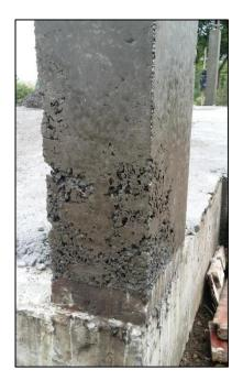
Fig.-2 Commonly Found Defect - Honeycombing
