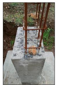
Fig.- 3 Improper Covering
