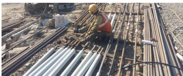
Fig 4.2 Anchor fabrication
