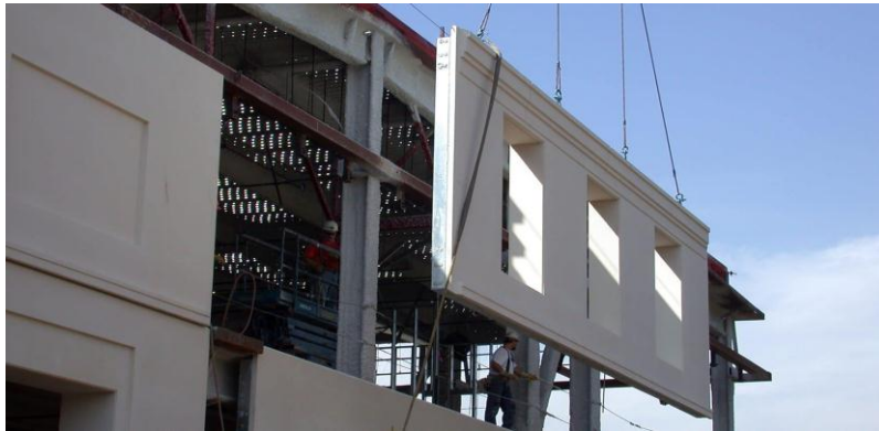
Fig. - 1: Precast construction ( https://theconstructor.org )
