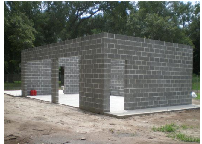
Fig-1.4: Hollow concrete blocks wall
