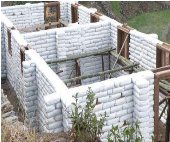
Fig-6: Earthen bag walls
