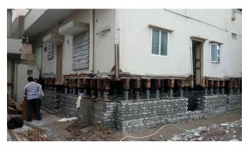
Fig. 1. Elevating house using Jacking Technology.
