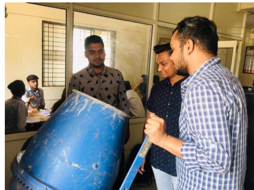
Figure 6 Mixing of concrete
