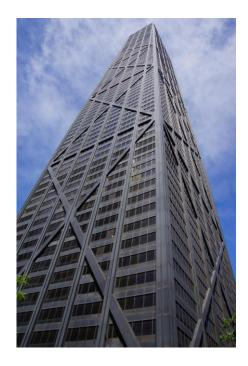
Fig. 3 Tube system in tall building.
