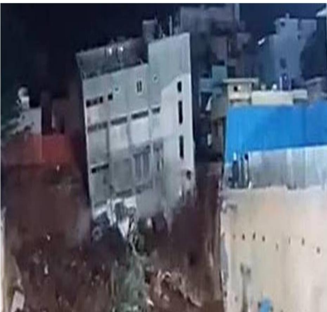
Fig. 7 collapse of apartment building Bangalore.
