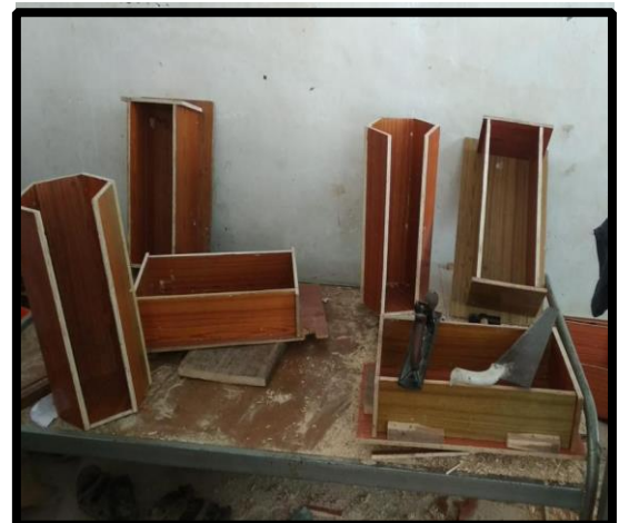
Fig. Formwork for different columns
