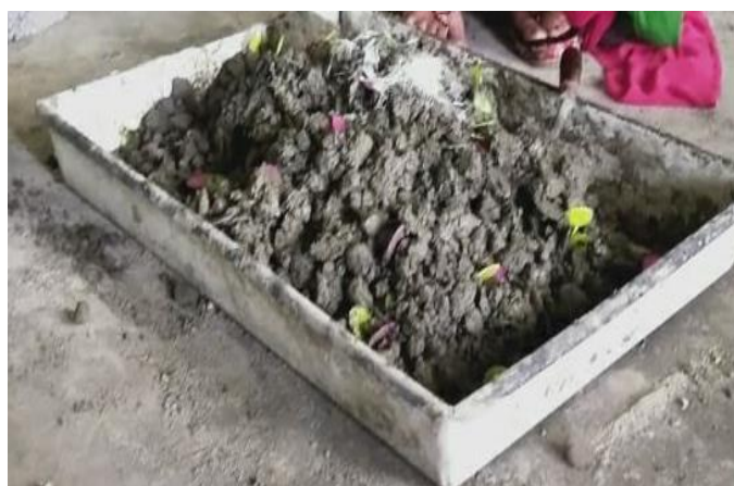
Fig.6 Mixing Of Concrete
