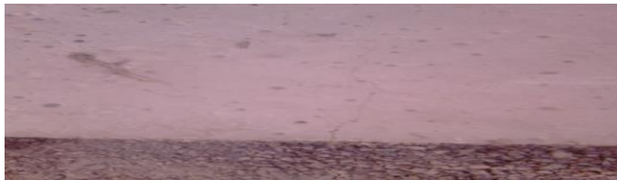
Fig. 10: First crack appearance for unreinforced beam
