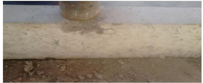
Fig. 14: First crack appearance for 2.0 % PFRC beam
