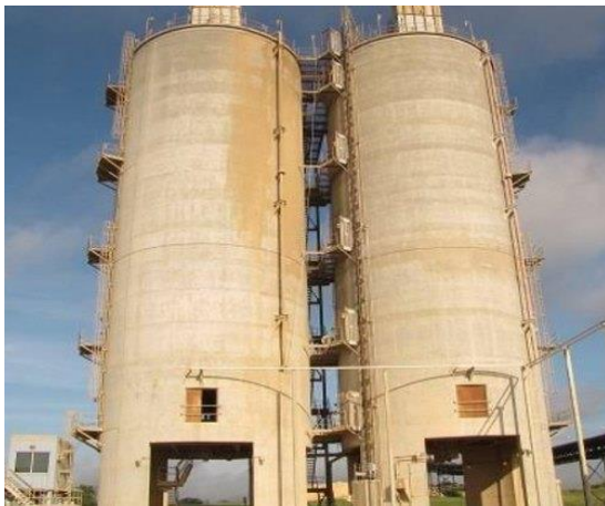
Figure 1: RCC Silo Construction
