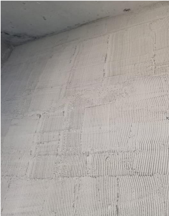
Fig 4.1- Eco Render+ application with V-notch trowel
