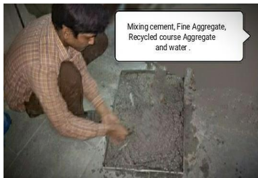
Mixing cement, fine aggregate (sand), recycled coarse aggregate and water.
