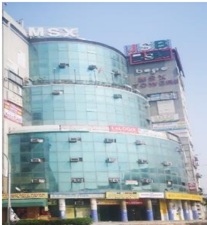
Figure 11. Building's facade, (Source: Author).
