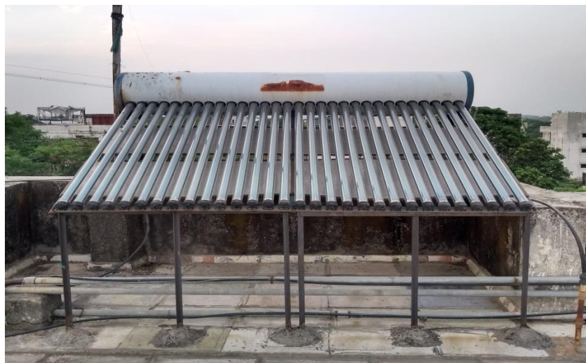
Fig – 1: A commercially available evacuated tube collector based solar water heater
