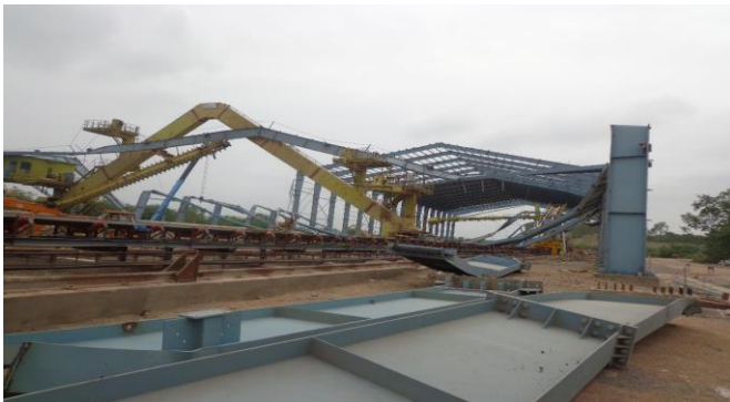
Fig. 8. Collapse of Wide and Tall Building along Ridge above Column Section Change
