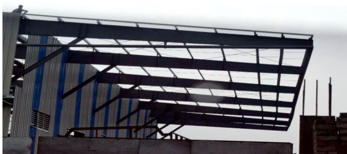
Fig. 5. Rehabilitation in Progress – Braces Added For Cantilevers
