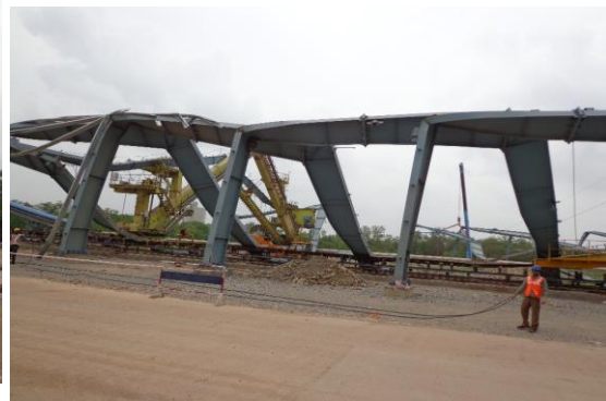
Fig. 8. Collapse of Wide and Tall Building along Ridge above Column Section Change
