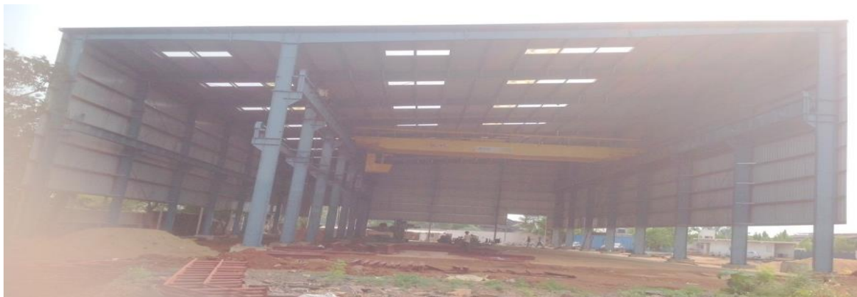
Fig. 13 Single Sloped Building Scheduled For Expansion – Deemed Failure
