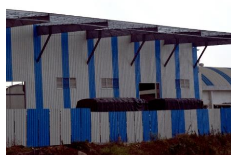
Fig. 5. Rehabilitation in Progress – Braces Added For Cantilevers
