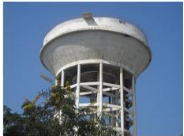
Fig 1: - Elevated intze water tank [11]
